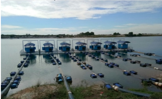
PUMPING OPERATION OF ALTERNATIVE PONDS (OPAK) AT BESTARI JAYA (800 MLD)
